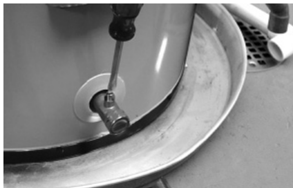
Figure 20 - Draining the old water heater.
