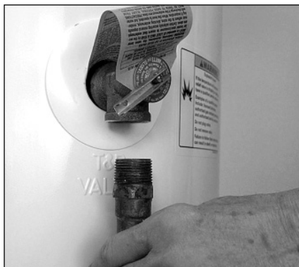
Figure 21 - Removing the T&P Relief Valve discharge pipe.
