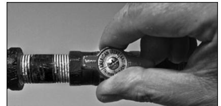
Figure 50 - Gas valve in "on" position.
