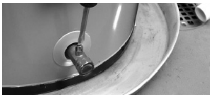
Figure 40 - Draining the water heater.
